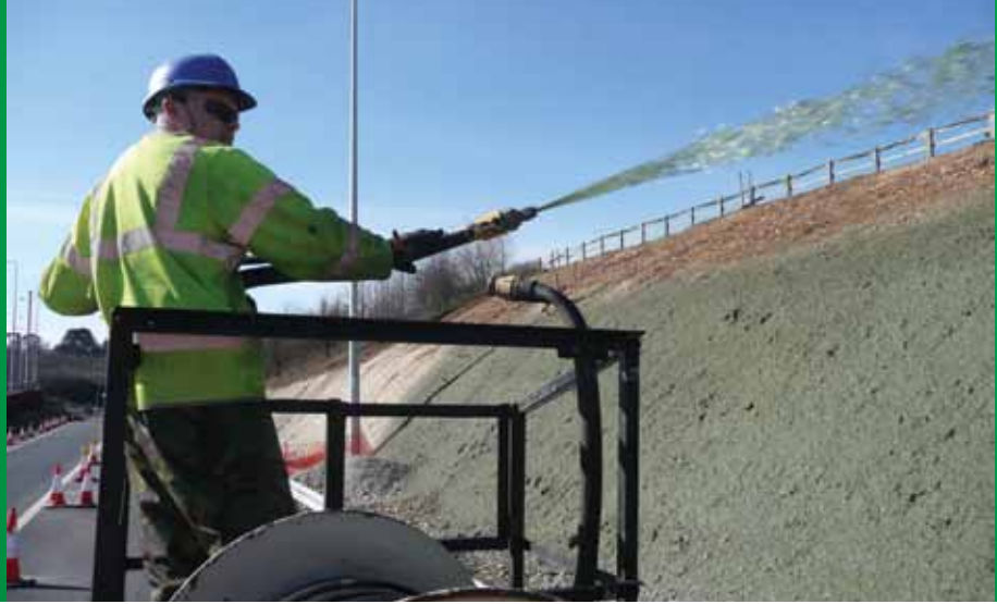
Slope erosion protection on the M25 Motorway, UK.
