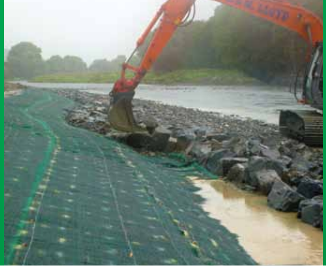
Riverbank protection works in mid Wales using VMax® P550, UK.
